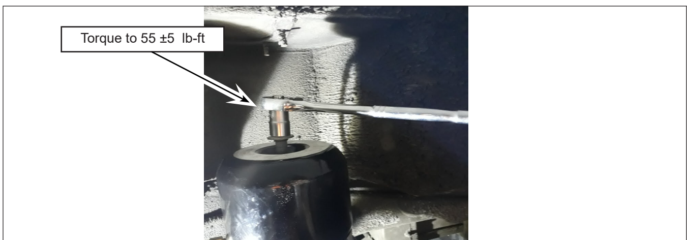
Figure 6 - Tightened the New Chamber Release Bolt
