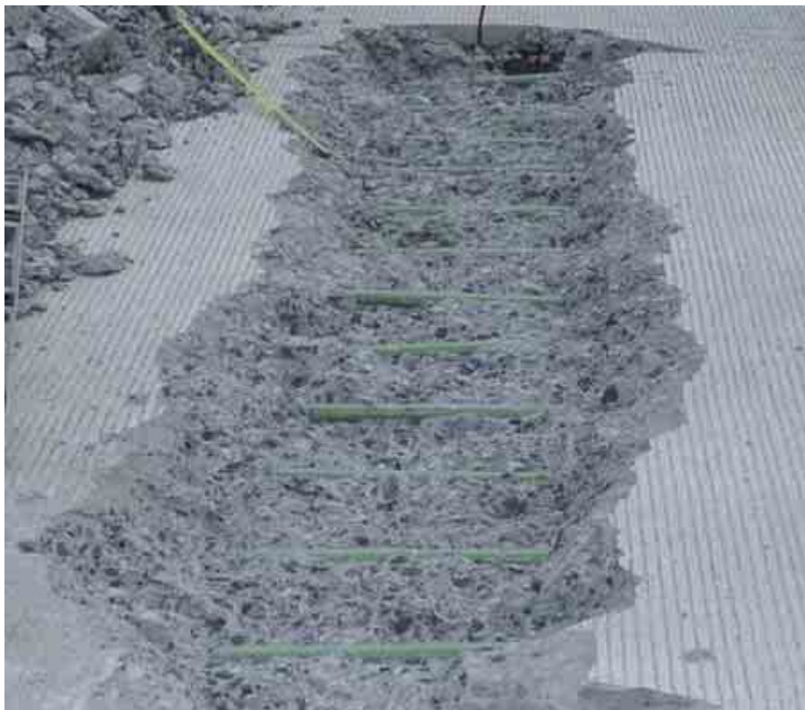
Figure 10. Exposed dowel bars for validation of MIT Scan-2 results.
